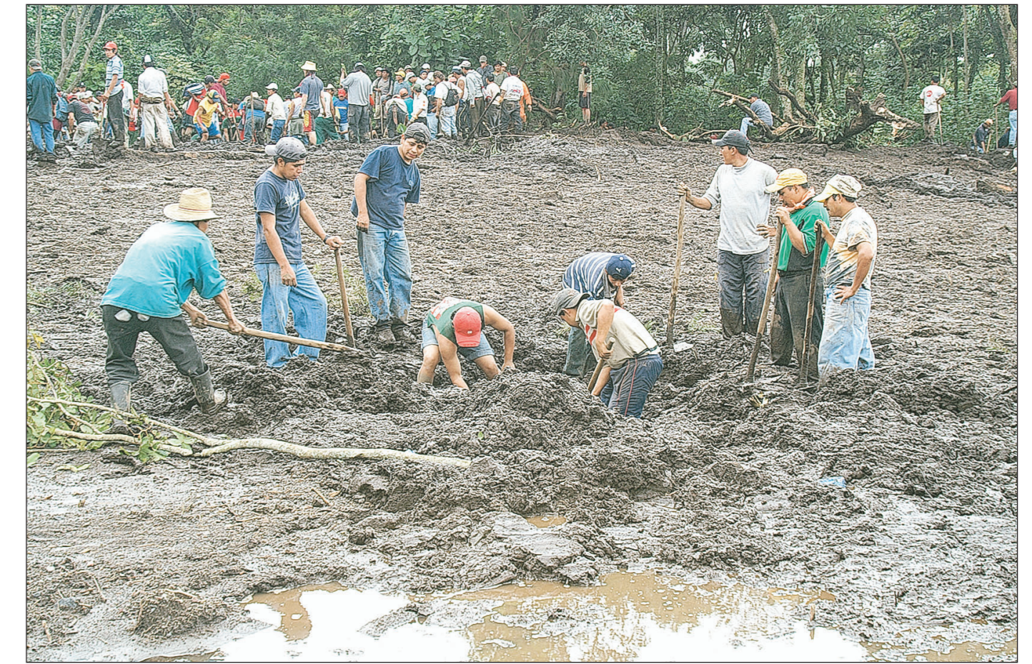
BELOW: Villagers and volunteers dig in the mud with farm implements as their only tools.
